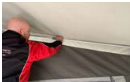
Attach the longer c-clip spreader bar
